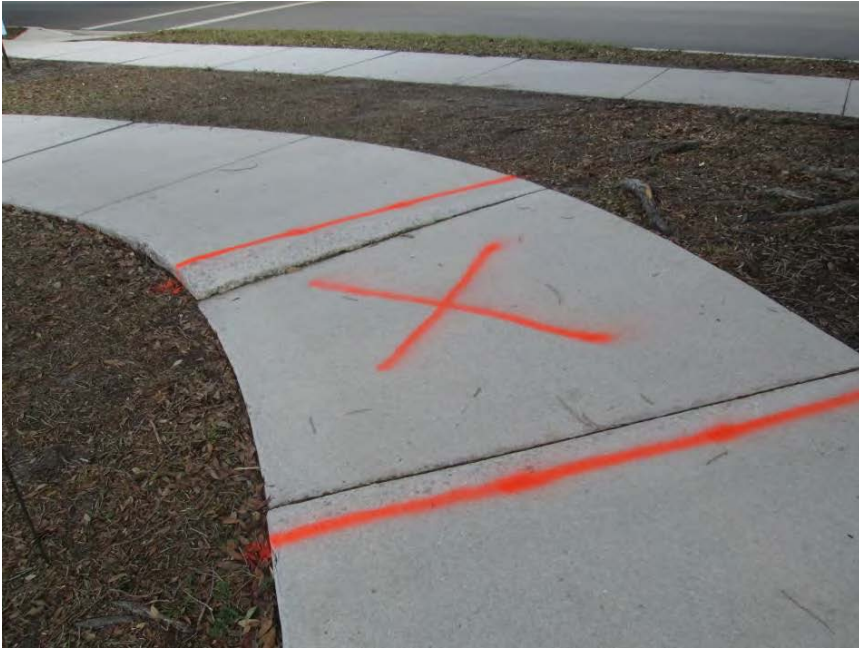
6.5' x 6' replacement near sports fields and Greyhawk Blvd
