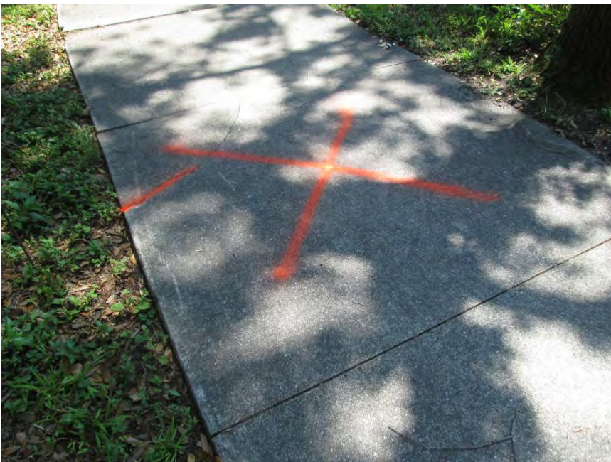
Remove & replace 5.5' x 6' at lot 19 Petrel Trail s/o Magpie
