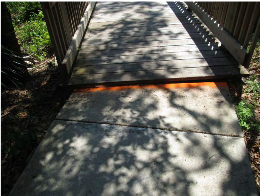
Remove & replace 2' x 5' wedge, add backfill under slab
