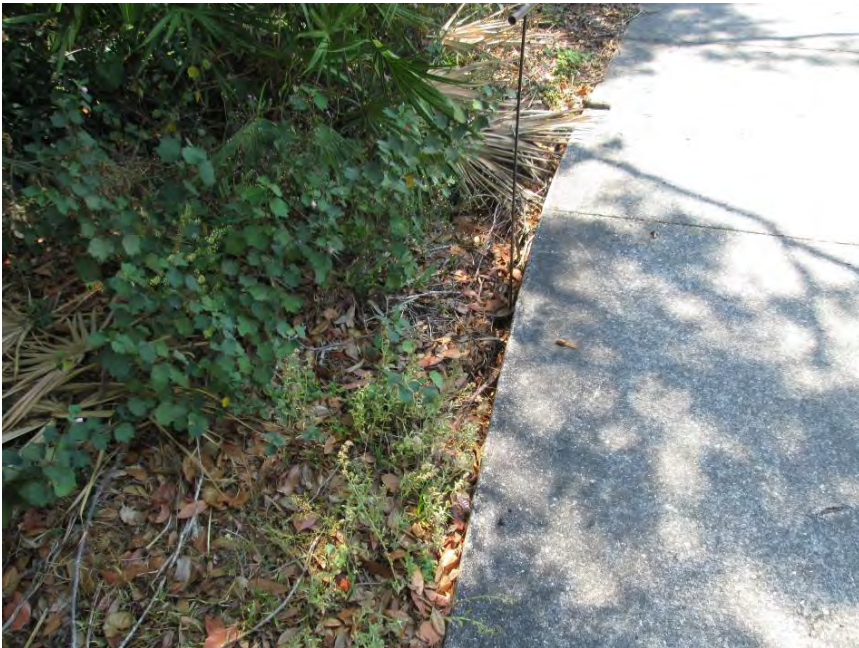
Add fill along east edge at lot 15/16 Petrel Trail
