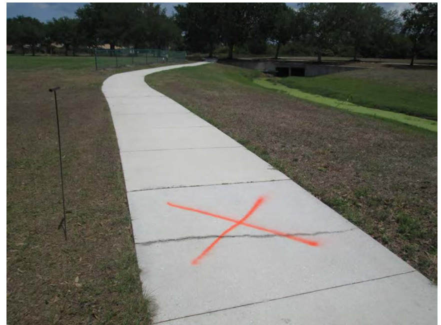
6' x 6' replacement near sports fields
