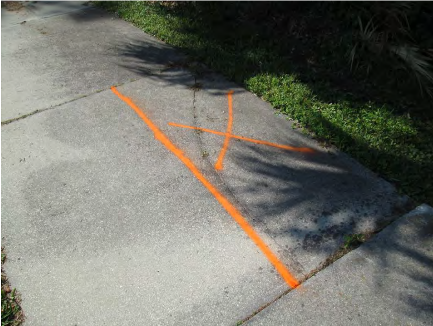
Remove & replace 6.5' x 3' section north of Daisy Place
