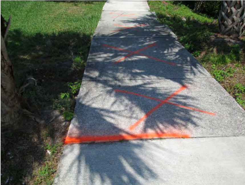
Remove & replace 22' x 6' at lot 18 Petrel Trail and add fill at edge
