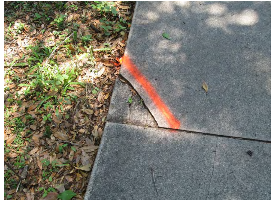
Remove & replace 18" triangle at lot 18 on Petrel Trail s/o Maggie
