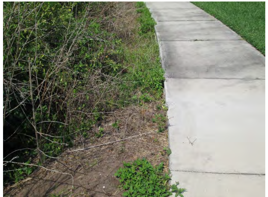
Add fill along edge +/- 30' at lot 281 Chantilly Trail
