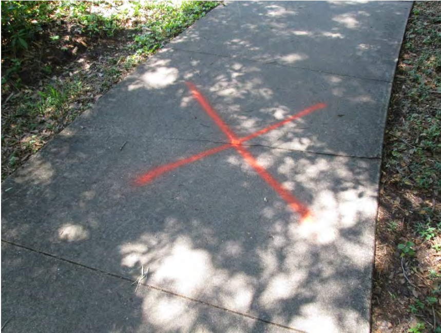
Remove & replace 7' x 6' at lot 18 Petrel Trail s/o Magpie
