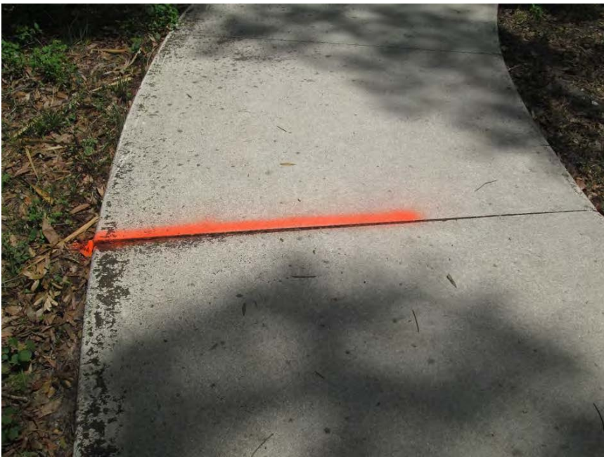
Grind on east side of Chantilly
