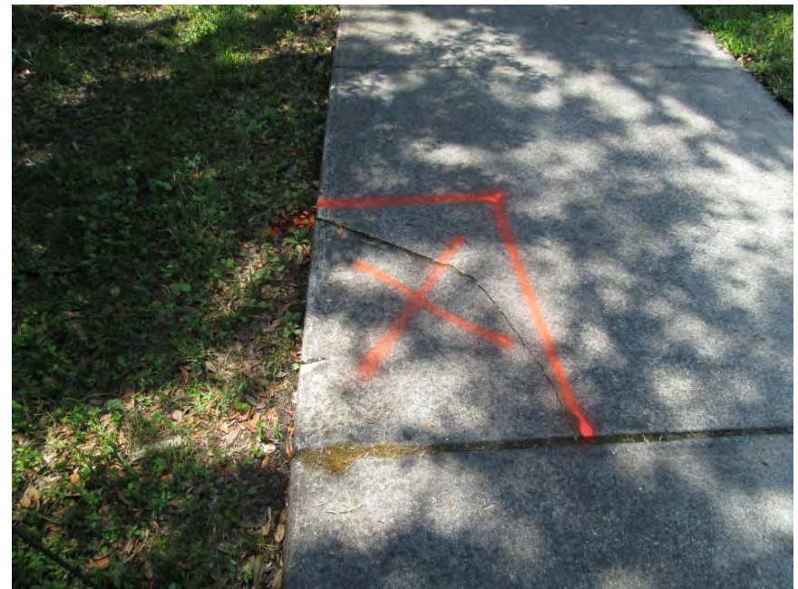
Saw cut and replace 4' x 2' section lot 27 Raven Terrace
